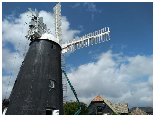
The Mill shutters were replaced in July
